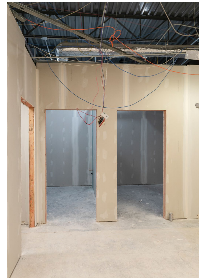
Interior construction progress of the new East End Clinic
