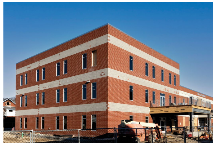
Construction progress on the new East End Clinic
